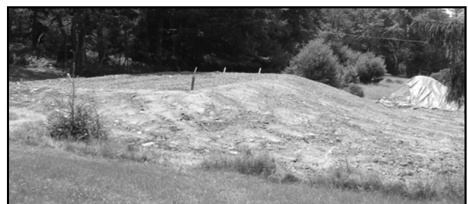
Sand Mound Under Construction
